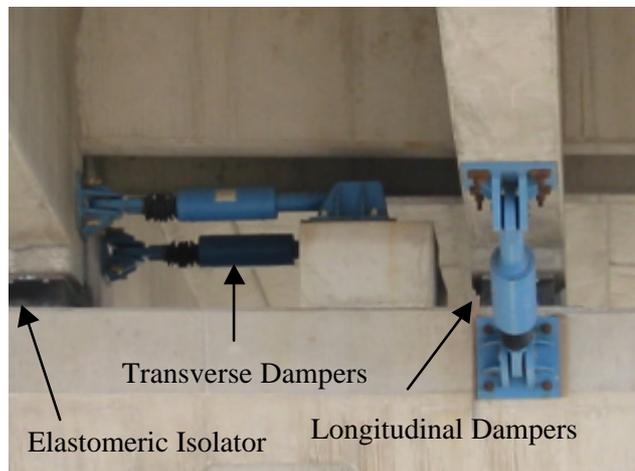
**Figure 6 – Isolation system in the Antirion approach viaduct.**
